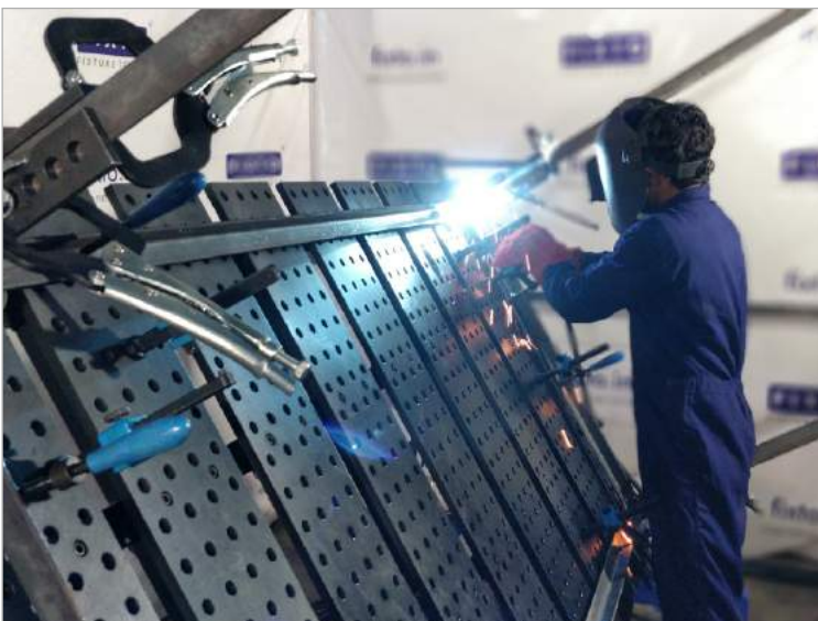
Welding in taper position
